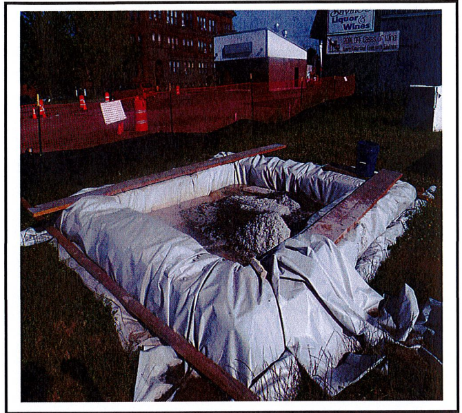
Concrete washout.
