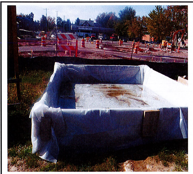
Concrete washout has been maintained.
