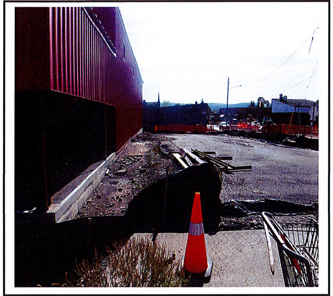
Future location of rain garden.
