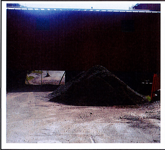
Soil is being stockpiled in the road.
