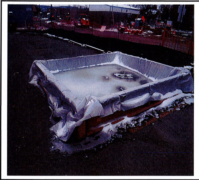
New concrete washout and new location.
