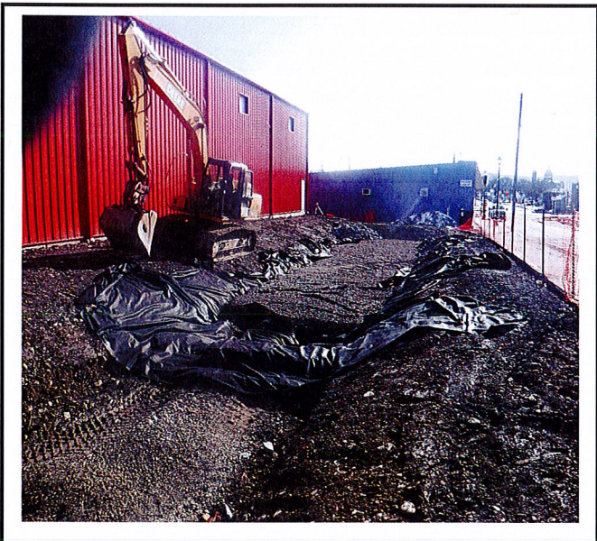
Rain garden is being installed.
