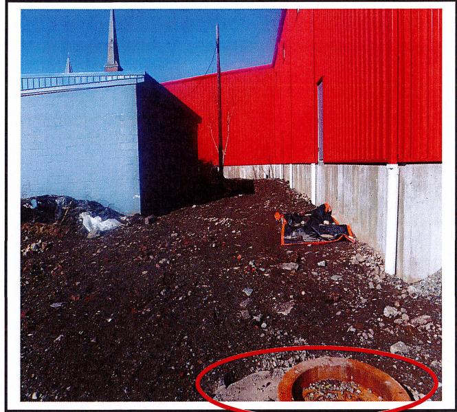
Manhole diversion structure lid open, soil can get into underground stormwater system.
