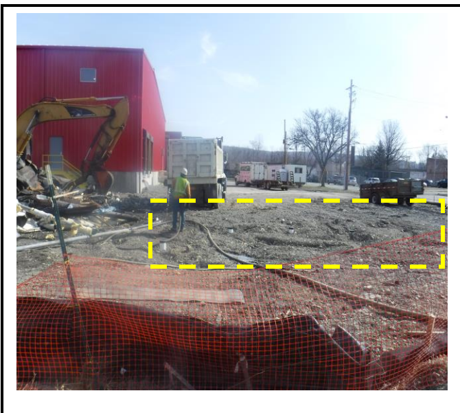
Dashed area represents the approximate location of the underground infiltration system. Dump truck hauling material out is directly on top of the system.
