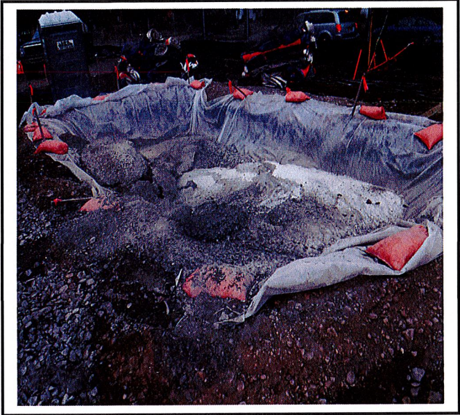
Concrete washout.
