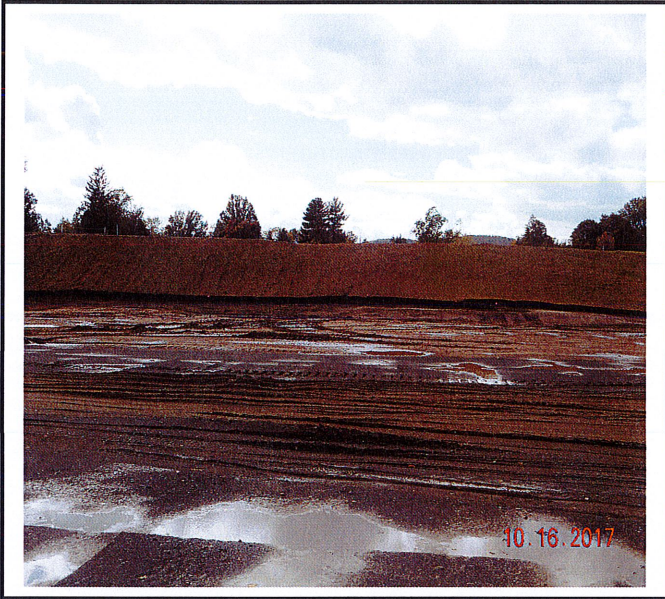
Soil stockpile has been stabilized.
