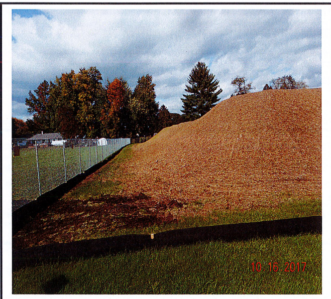
Stockpile has been stabilized and has filter sock surrounding it.
