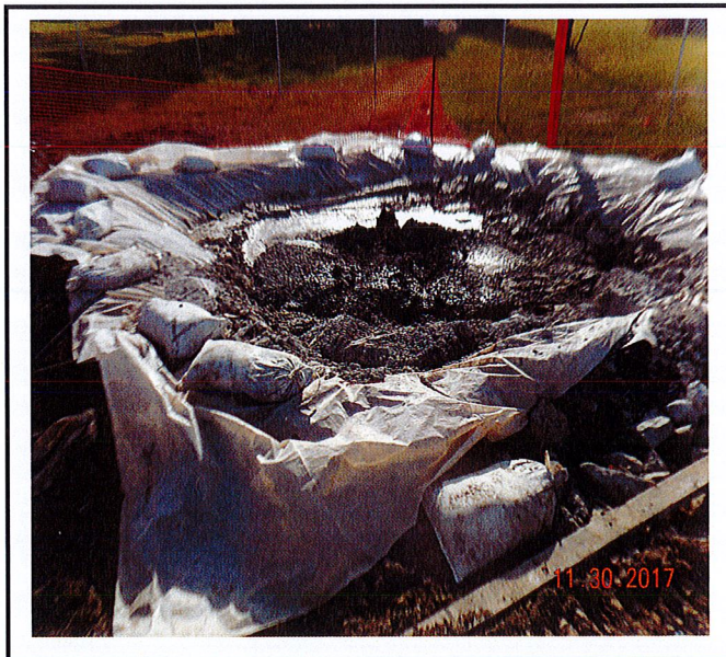
Concrete washout installed and being utilized.
