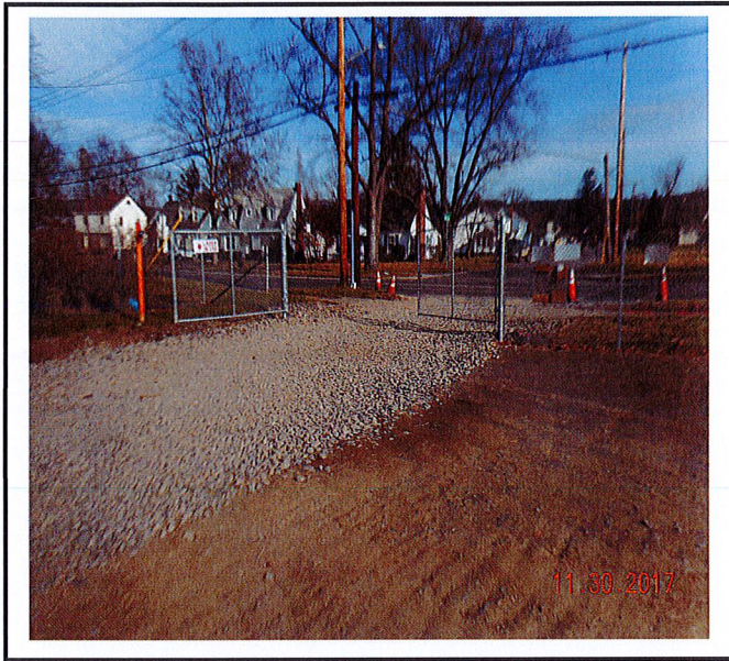
Construction entrance in good shape.
