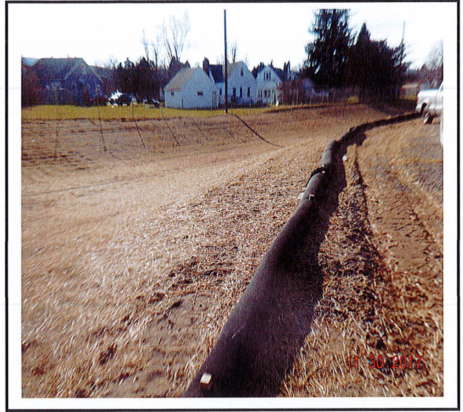
All areas have been stabilized.
