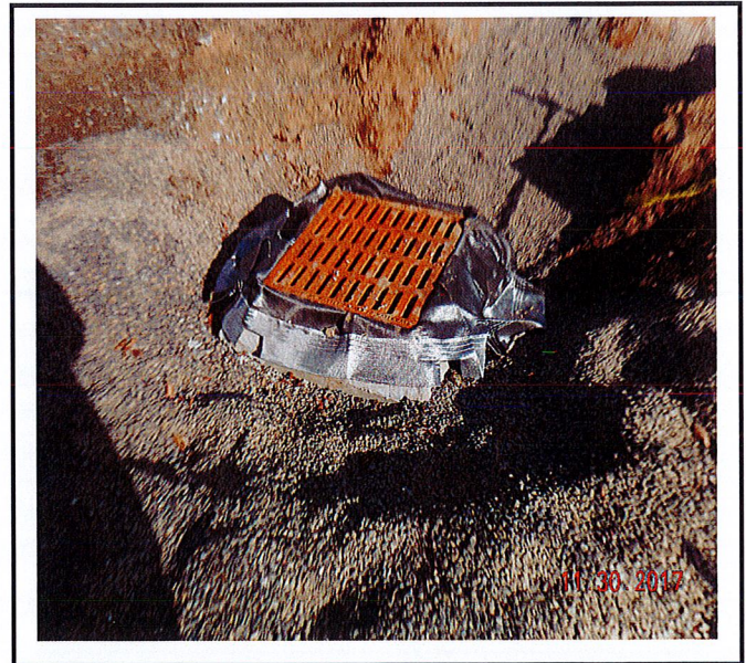
All catch basins have inserts and are protected.
