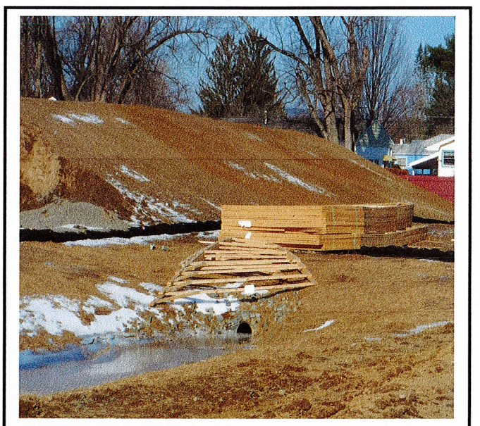
Roof trusses stored on top of the compost sock.
