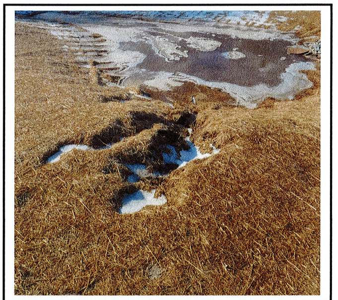
Active erosion occurring in forebay.
