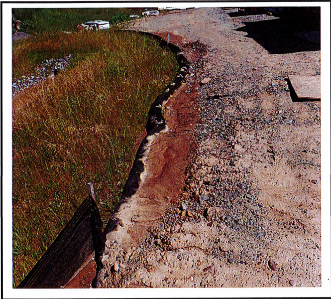
Compost sock at the rear of the building is over capacity and needs replacement or silt needs to be removed .
