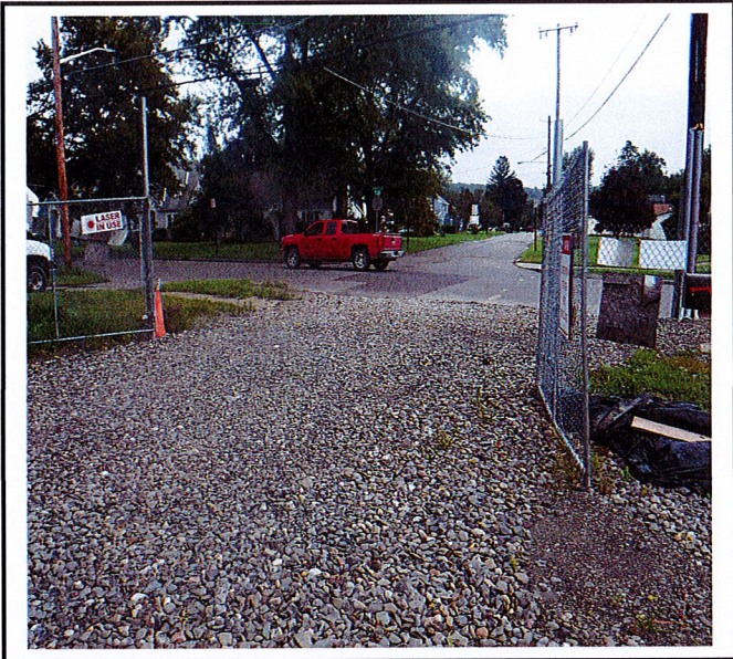
Construction Entrance is in working condition.
