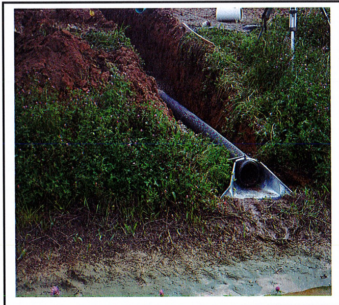
Roof drain line to west forebay.
