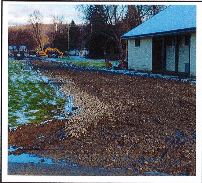
Construction road at rear of project.
