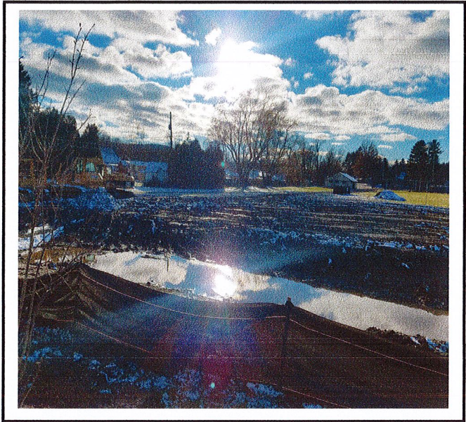
Standing water in forebay.
