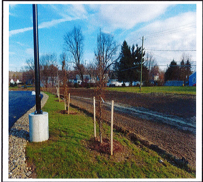
Infiltration basin has been re-graded during high soil moisture.
