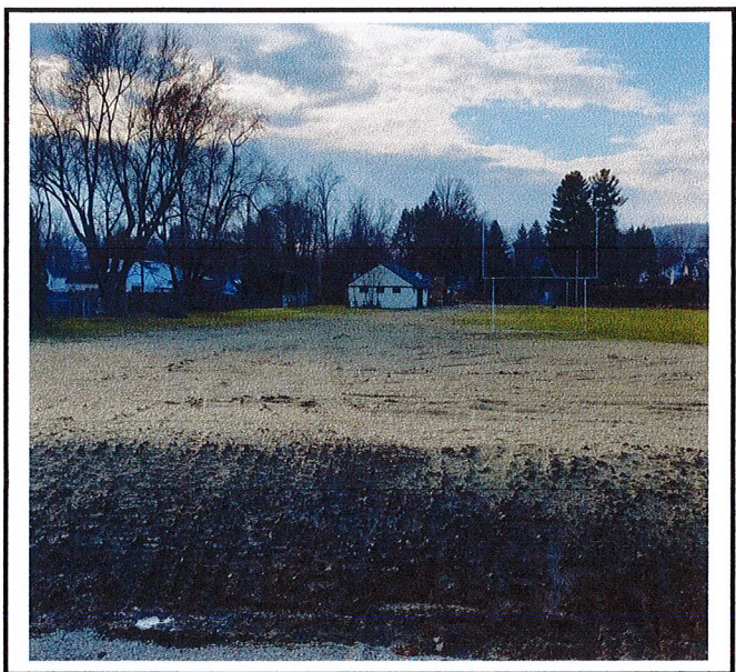
Stockpile and staging area has been graded and stabilized.
