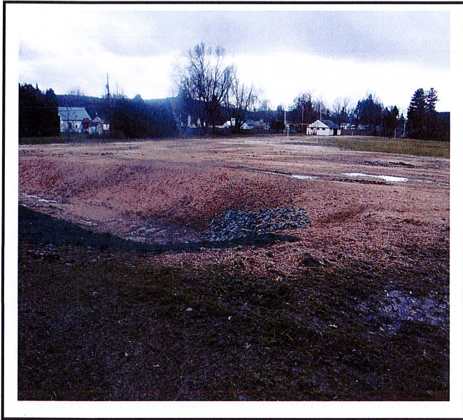
All open soil has been covered with blankets or mulch.
