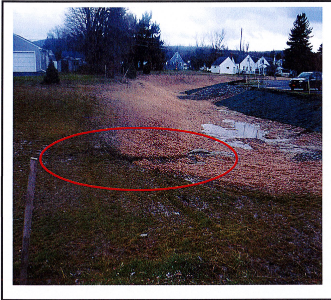
Erosion from front lawn is occurring from surface runoff.
