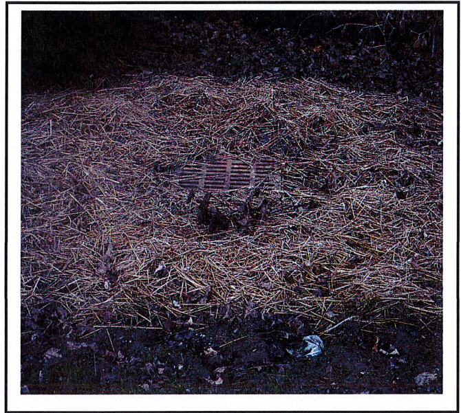
Inlet protection has been removed around catch basins.
