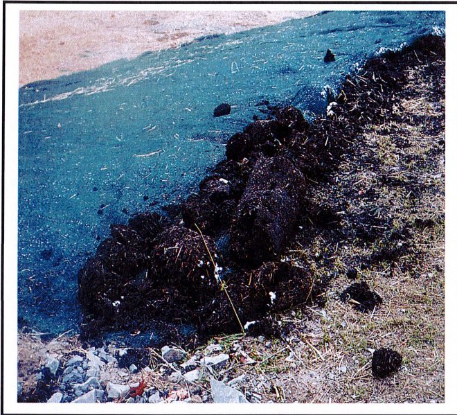
Compost sock removed but mulch not removed or raked flat.
