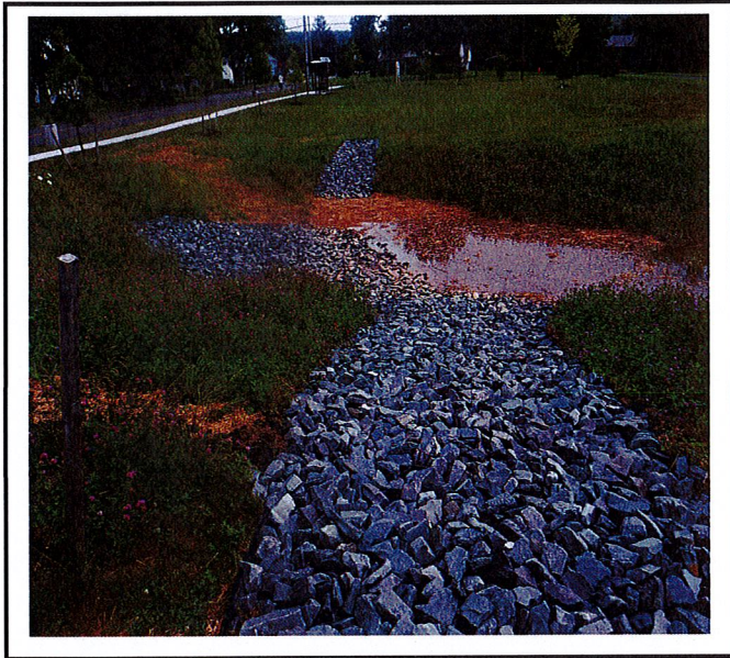
Rock added to the areas that had runoff and erosion issues.
