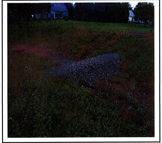
Stone berms have been repaired.
