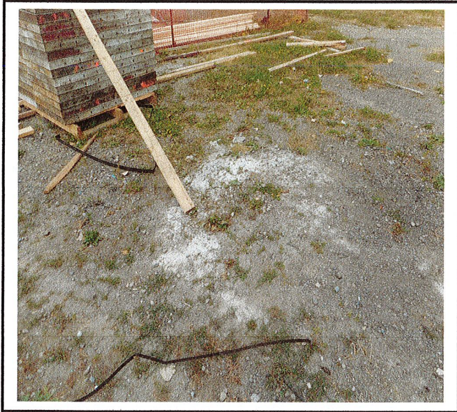
Concrete washed onto ground.
