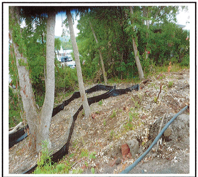
Double row of silt fence installed.
