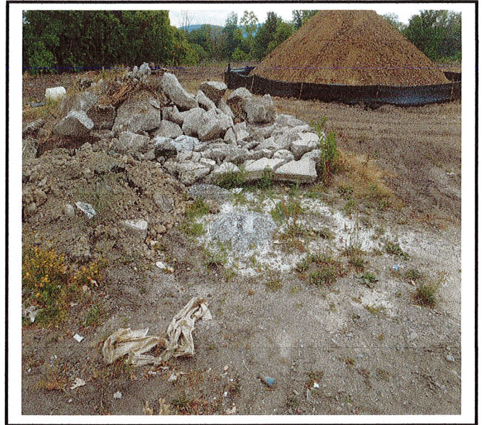
Concrete washed onto ground.
