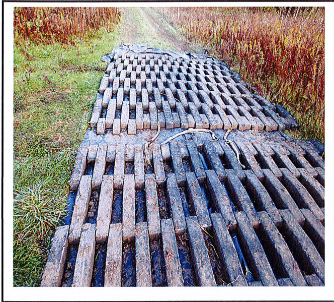
Mats used as a construction entrance.
