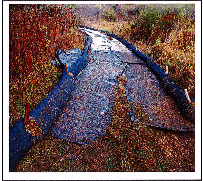
Mats used as construction entrance.
