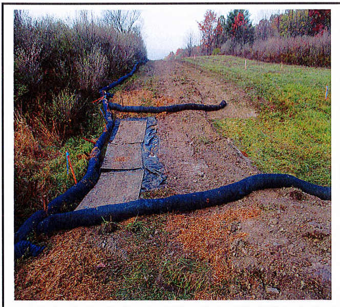
Silt socks installed at all planned locations.
