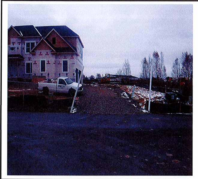
Construction entrance to Lot #85.
