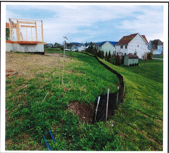
Silt fence requires repair.
