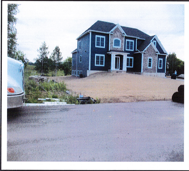
Lot 85 prepped for sod stabilization.
