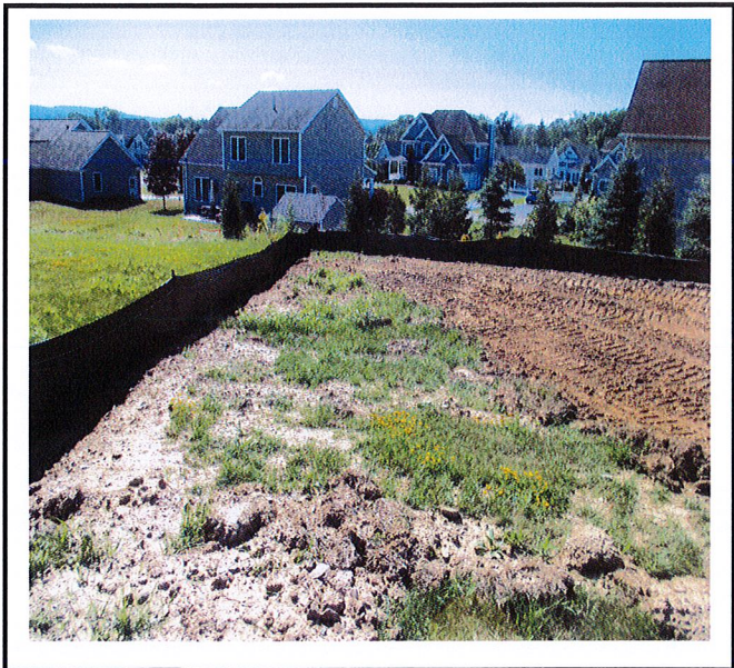
Erosion controls are in place and functioning.
