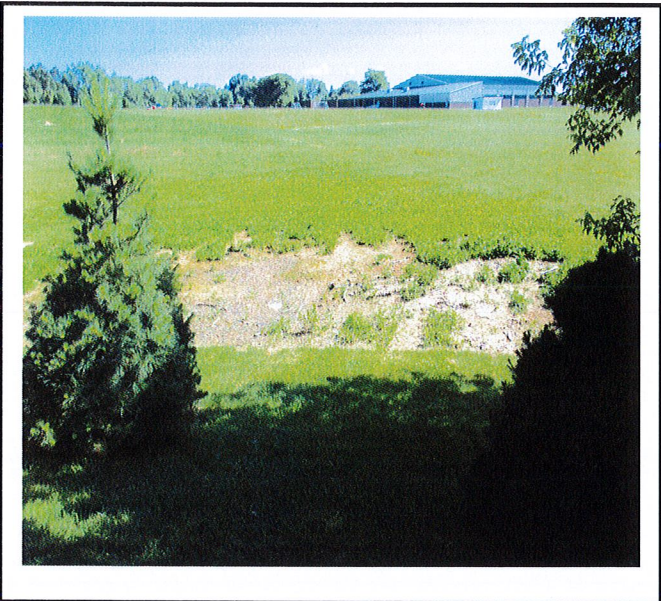
Area where stormwater goes onto school property and pools.
