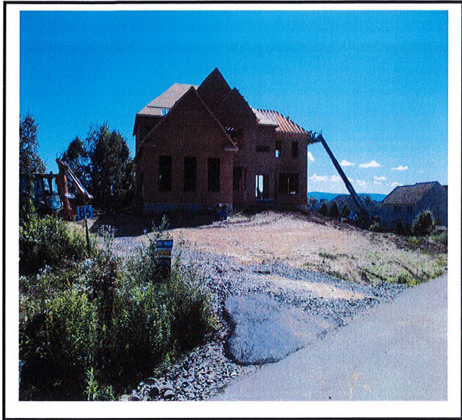
Lot 86 is under construction.
