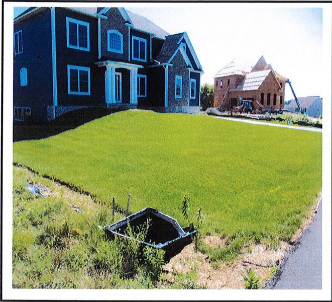
Lot 85 is now stabilized.
