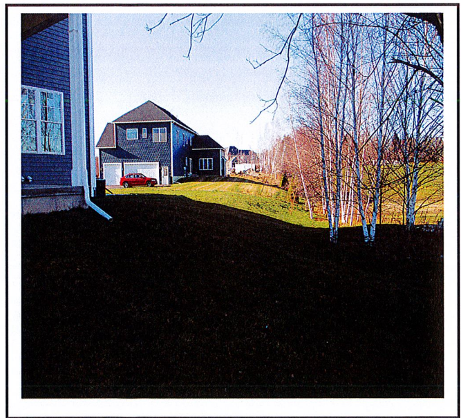
Backyards stabilized of lots 85 and 86 completely stabilized.
