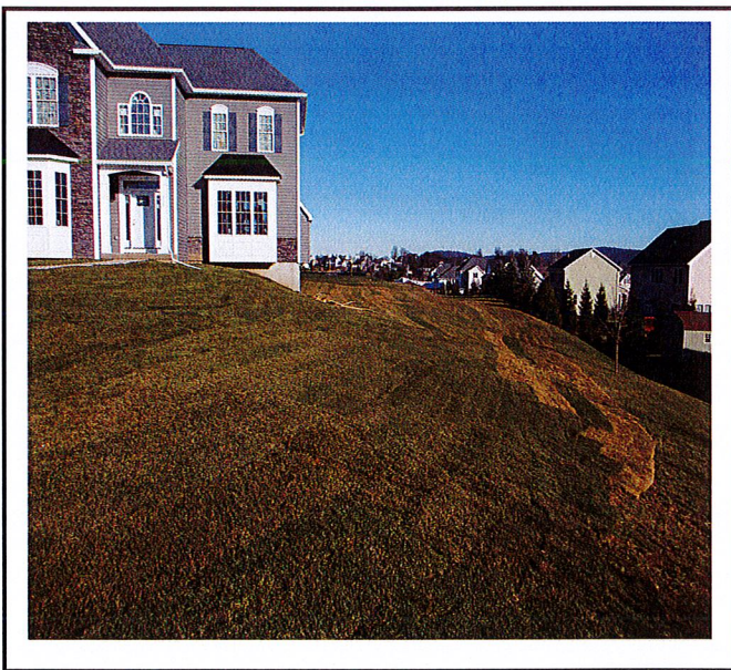
Lot 86 completely stabilized.
