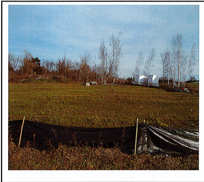
All soils stabilized and silt fence functioning.
