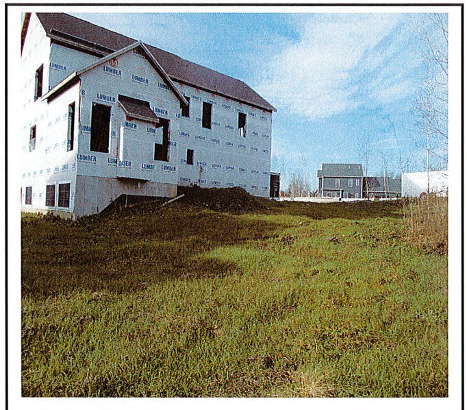
All soils have been stabilized.
