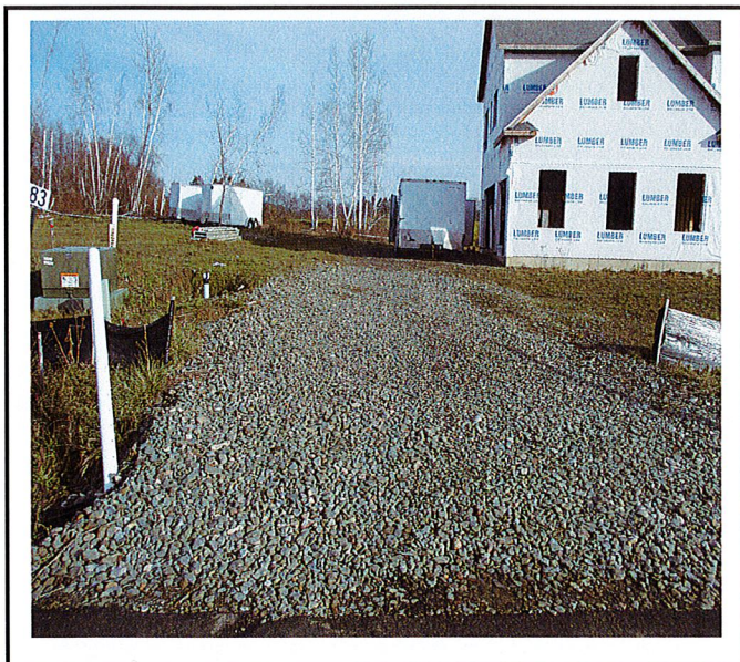
Construction entrance in good shape.
