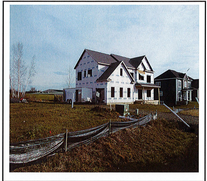
All soils stabilized and silt fence functioning.
