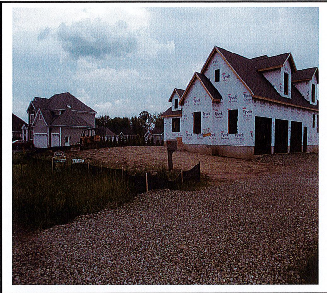
Construction entrance in working order.
