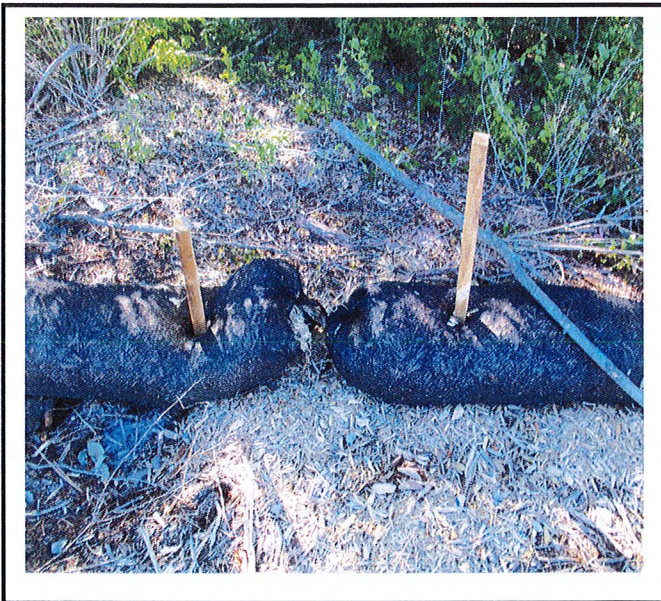
No overlap on the compost filter sock.
