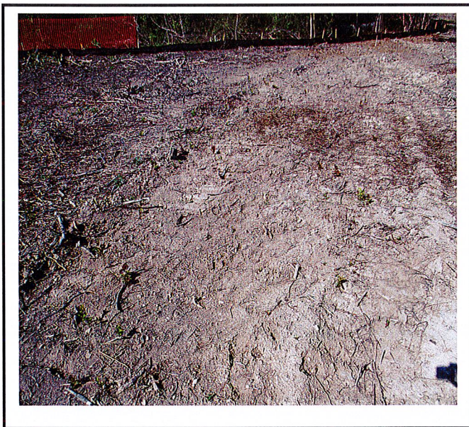
Some areas have no soil stabilization.
