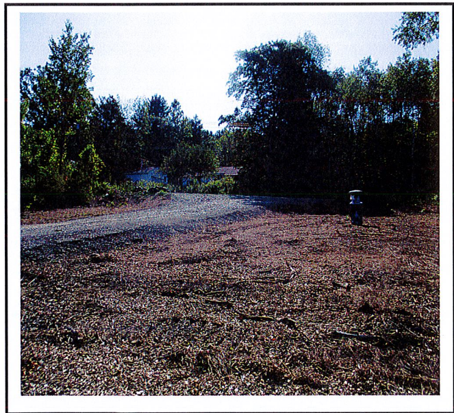
Construction entrance is in good condition.
