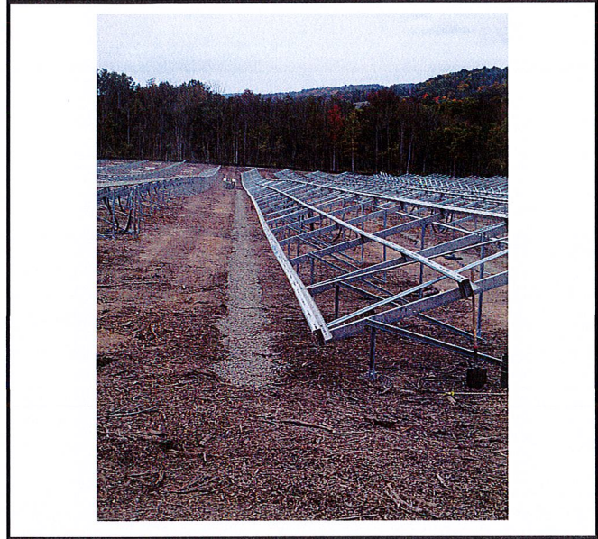
Flow diverters are being installed where they are planned.
