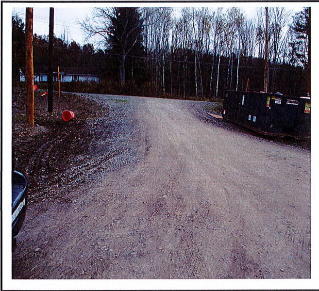
Construction entrance in okay shape but will need fresh stone soon.
