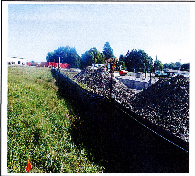
Silt fence has been installed around the perimeter.
