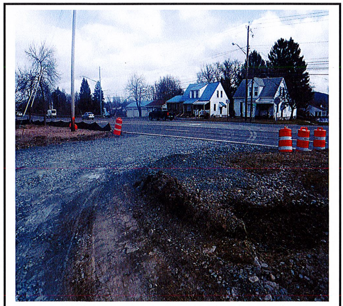
Construction entrance in good shape.
