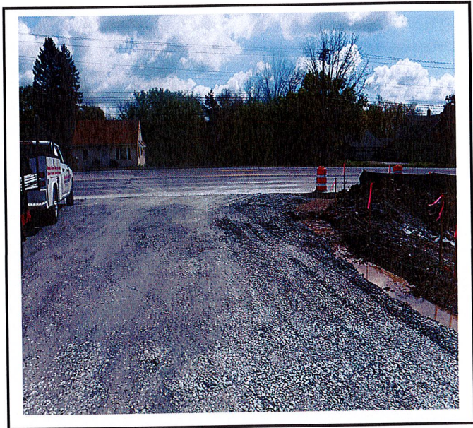
Well maintained construction entrance.
