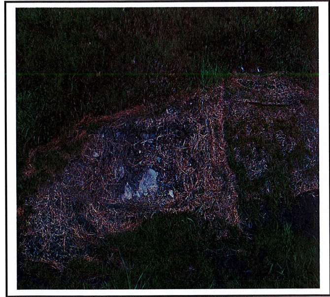
This is the drainage swale on the back side of the property. The slope on the left should be monitored. It looks like erosion could occur.
