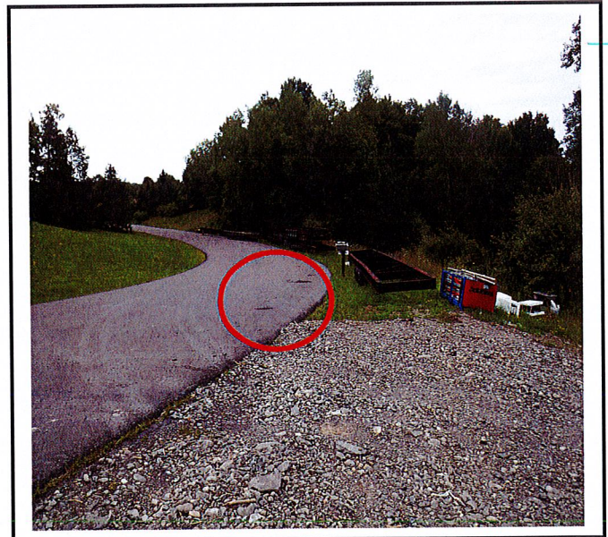
Stains from leaking equipment left on the road.
