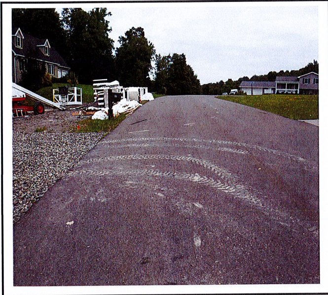
Garbage and debris stacked in municipal right of way.
