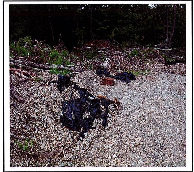
Garbage/construction debris strewn across the site.
