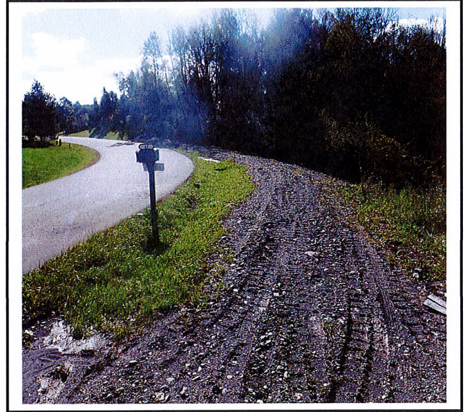
Sullivan trail has installed gas line.
