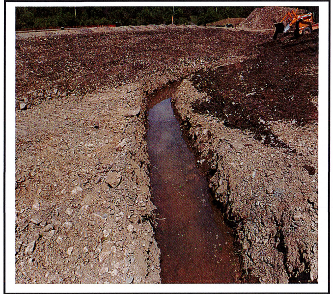
Low Flow Channel for the infiltration basin is filled with water. There is a minimum separation between infiltration practices and groundwater.
