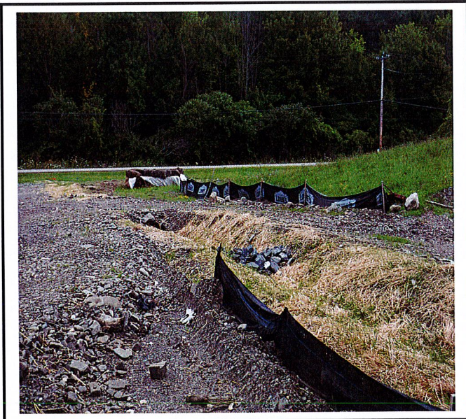
Drainage swale has been seeded and mulched as requested.
