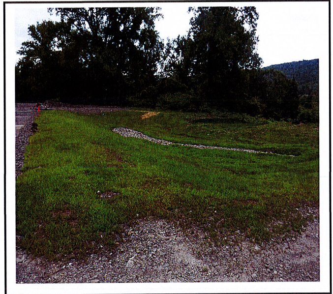
Infiltration basin is growing grass.
