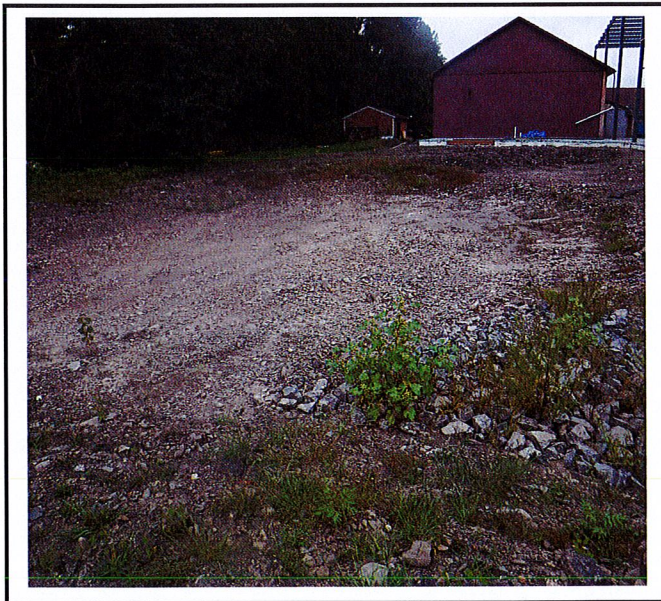
Temporary sediment trap/future stormwater forebay.
