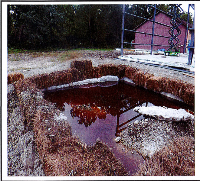
Concrete washout
