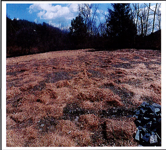
Former location of topsoil pile. Area has been mulched but it is no longer covering the entire area.
