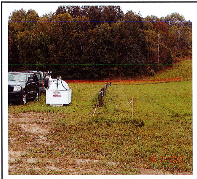
Silt fence installed.
