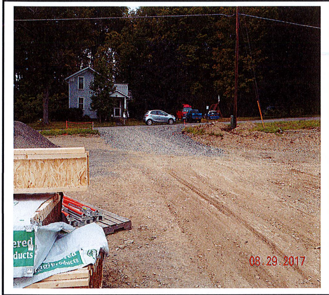
Construction entrance installed.
