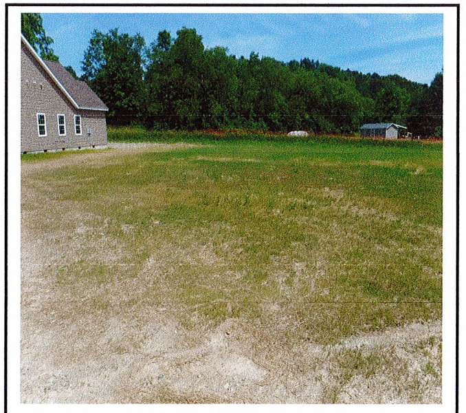
Grass growing in areas that have been temporarily stabilized.
