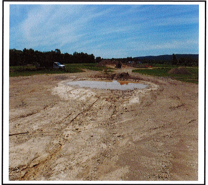
Sediment trap constructed in road area.
