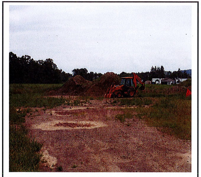
All soil/gravel stockpiles have been seeded.
