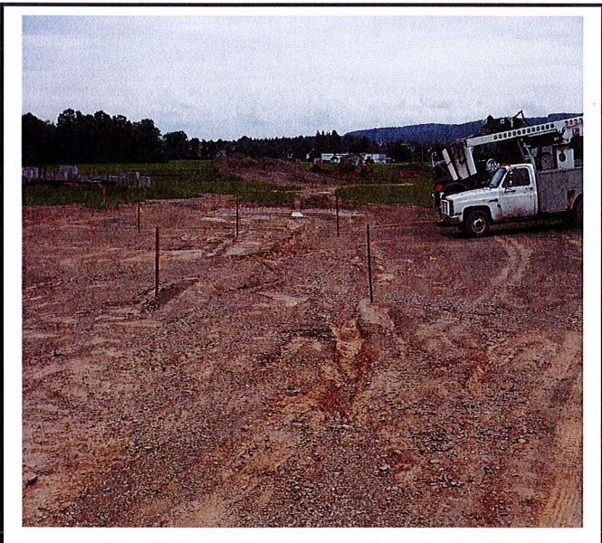
Temporary driveway runoff flows to a makeshift temporary sediment trap.
