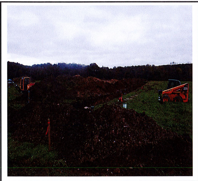
Water line is being installed.
