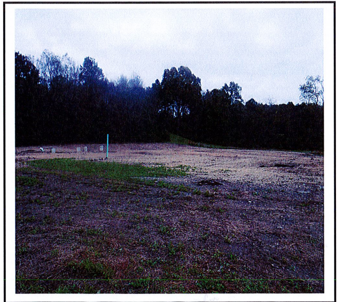
Septic field has been seeded and mulched.
