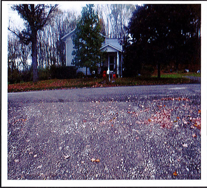
Construction entrance functioning.
