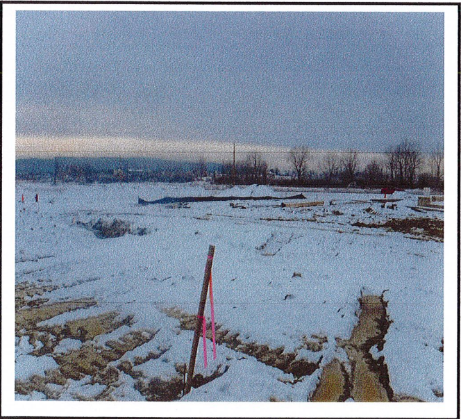
Overview of site.
