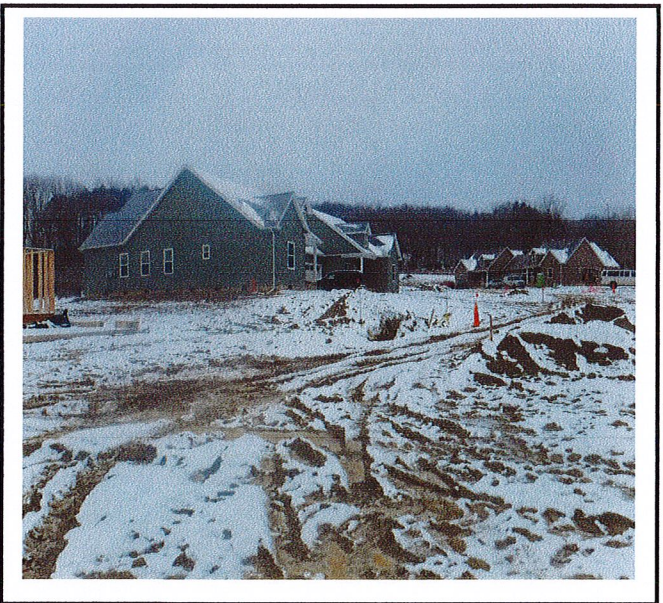
Overview of site.
