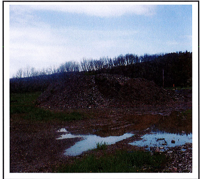
Topsoil pile requires stabilization.
