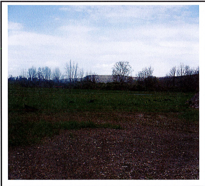
Silt fence needs to be replaced.
