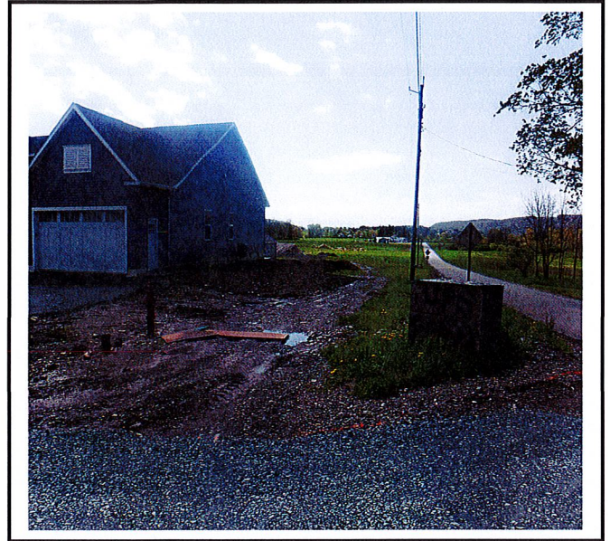
Topsoiling has started in preparation of stabilization with seed and mulch.
