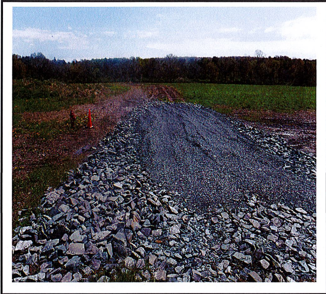
Additional construction entrance has been added.
