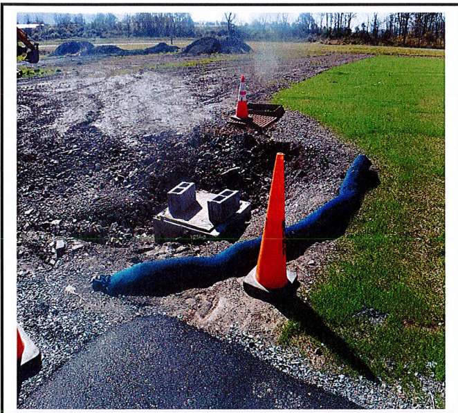
Storm sewer and catch basins are being installed.
