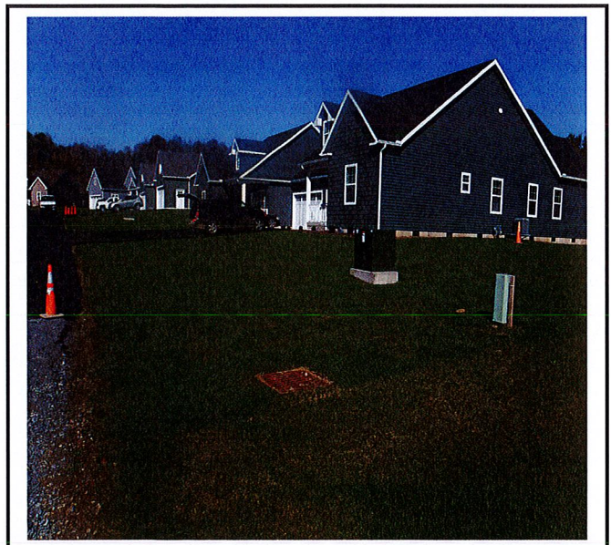
Areas around the houses have been stabilized.
