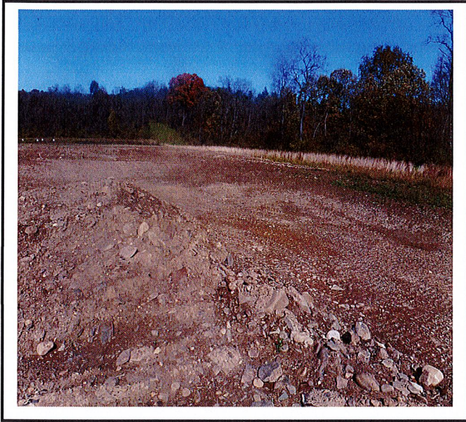
Stormwater basin under construction.
