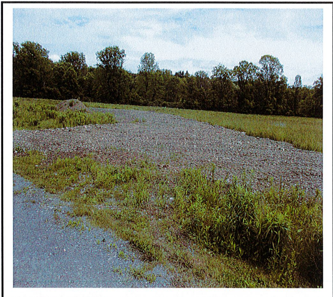
Open bare soil will need to be stabilized.
