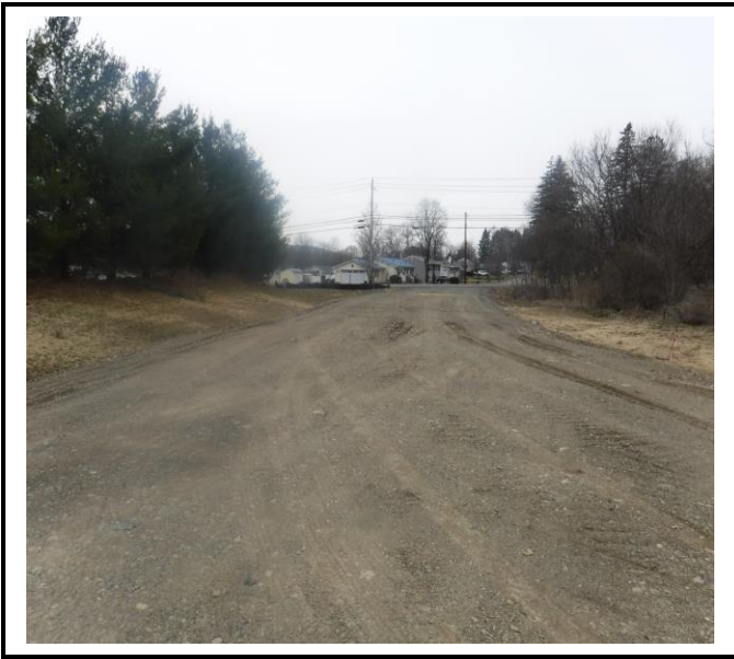
Construction entrance is working order.
