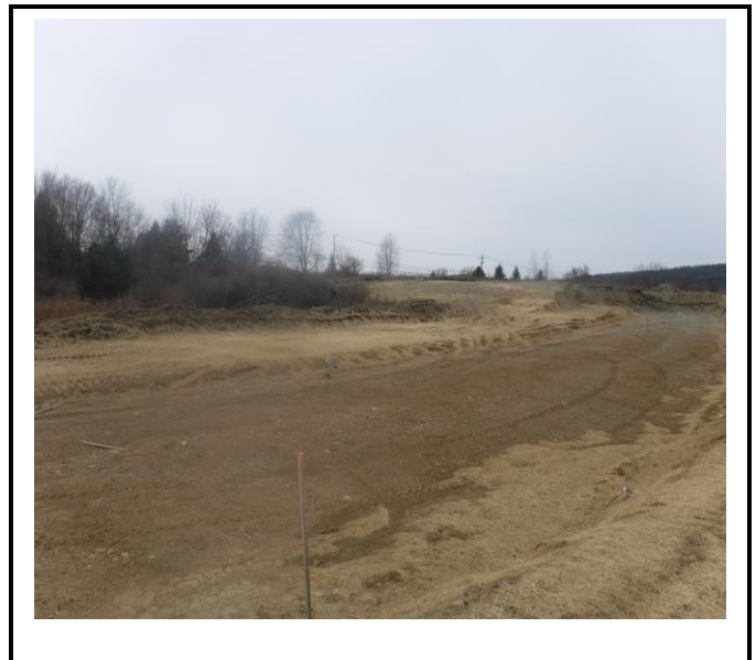
All open soil, except the house, has been stabilized.
