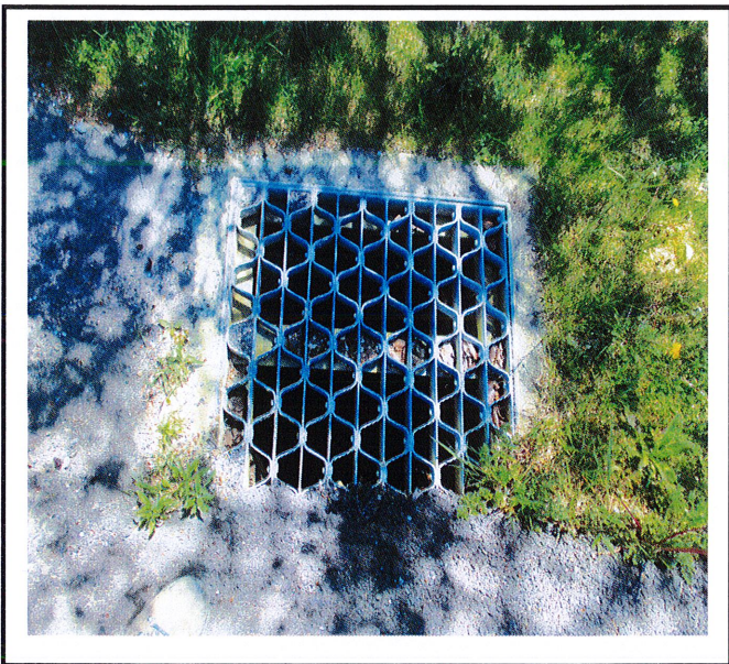
Catch basins have been cleaned off since last inspection.
