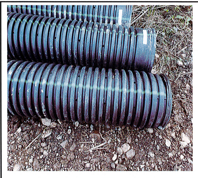
Storm sewer pipe for installation. Smooth interior and perforated as designed.
