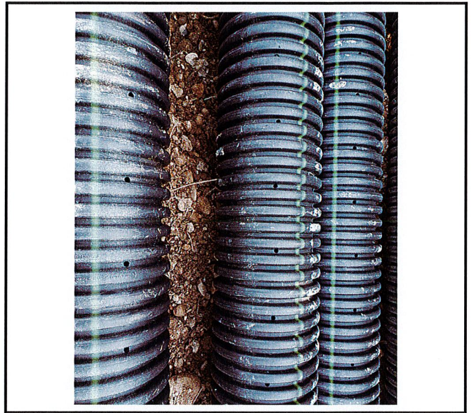
Storm sewer pipe for installation. Smooth interior and perforated as designed.
